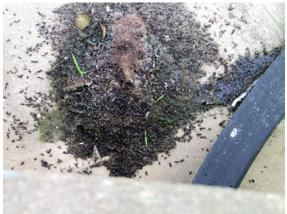
Photo 3: Example of open concrete joint used by bats Photo 4: Guano deposits visible from bridge deck, on top of pier
